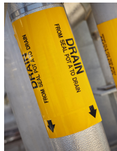
PIPE MARKERS PLACED IN HVAC INSTALLATION
